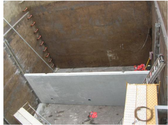
Figure 2: Installation of prefabricated partitions
