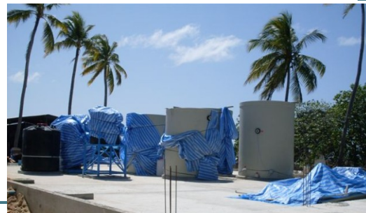
Aqwise new under construction Package Plant in a Pacific island
