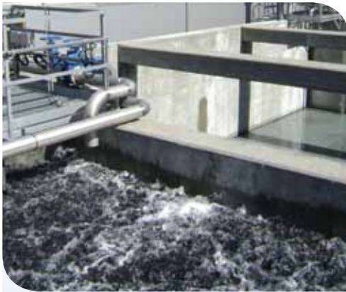
Paper mill, Greenfield–Portugal (1,200 m 3 /d)
