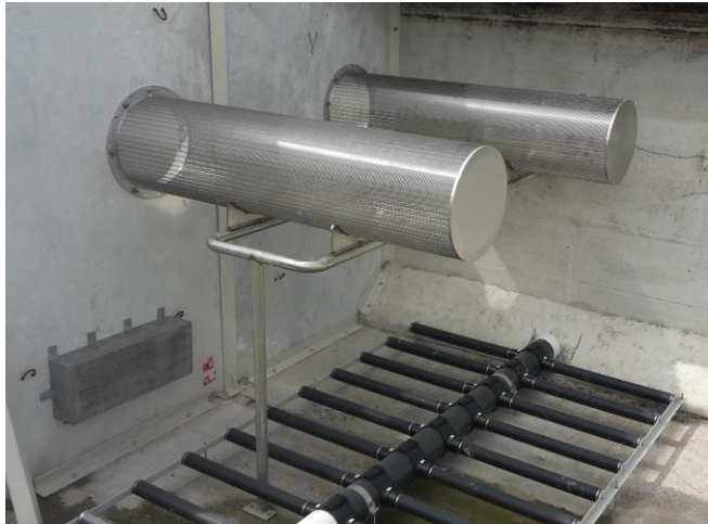
Figure 5. Installation of fine bubble diffusers and retention screens
