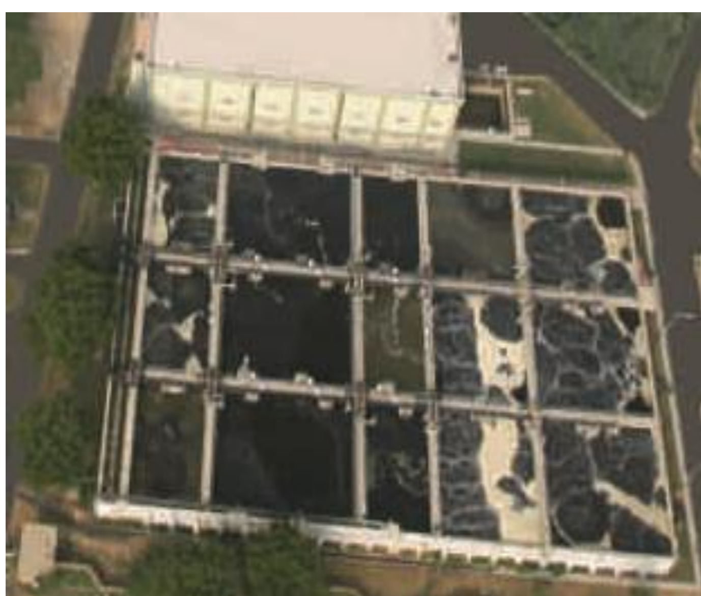
Figure 2 – Aerial view of the MBBR reactor
